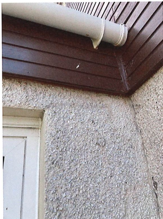
External -west extension wall – high level crack
