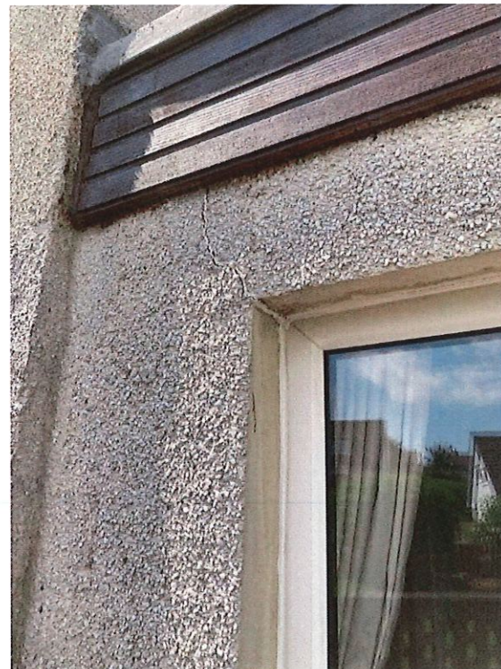
External -east extension wall – high level diagonal crack
