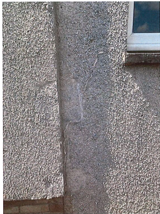
External – east extension wall – cracks in render Infilled with sealant.
