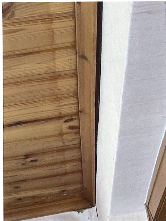
Extension – timber ceiling – gap at join with main house
