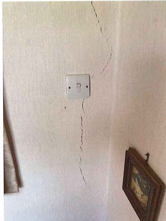
Extension – cracks in right hand east return wall – close up
