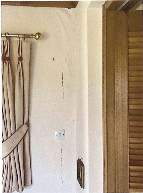
Extension – cracks in right hand east return wall
