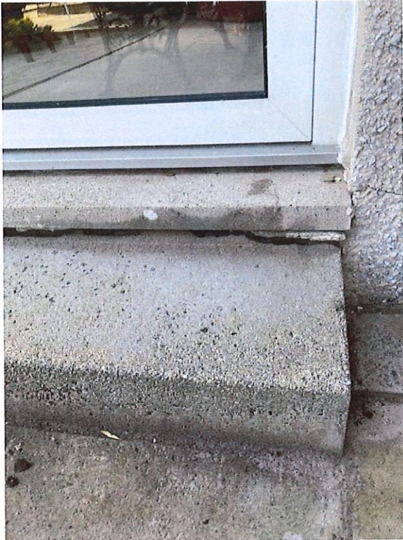
External -west extension wall – step has settled away From threshold.
