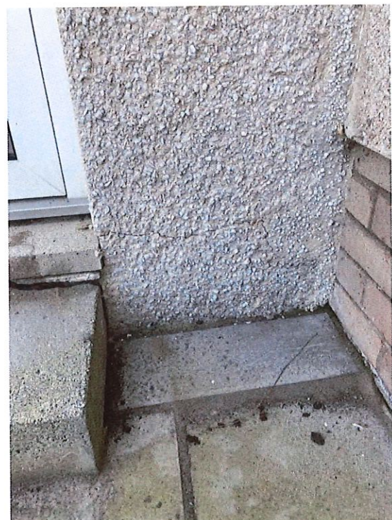
External -west extension wall – low level crack
