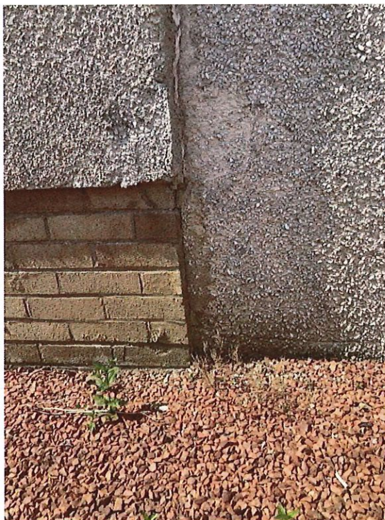
External -east extension wall – low level crack
