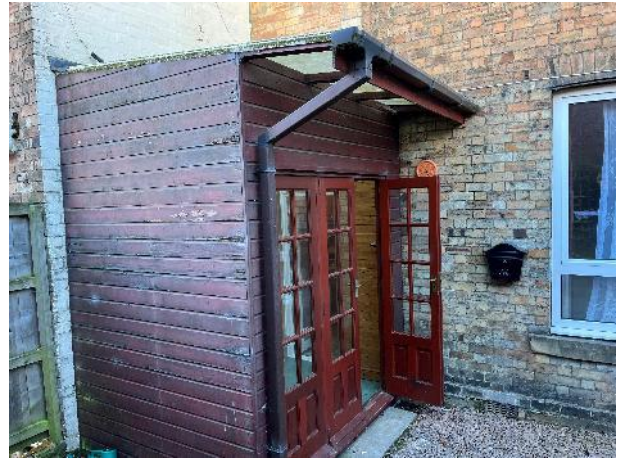
Rear timber porch
