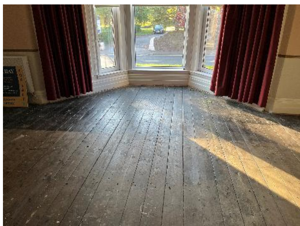
Front bay window – internal
