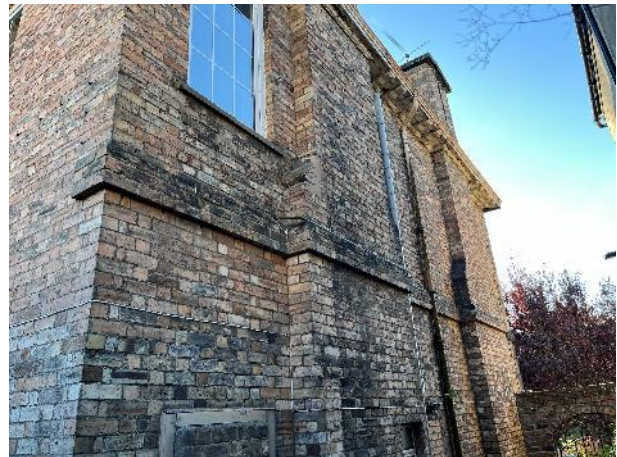
Chimneys on gable
